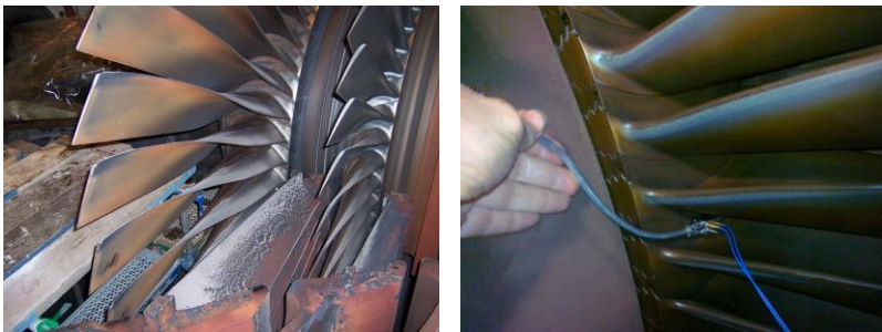
Figure 1.42 Left: blades in place. Right: UT-PA inspection of fir tree
