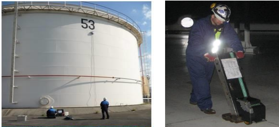
Figure 1.11 Mechanized inspection techniques of storage tanks. Left: wall thickness measurement using a 'crawler'. Right: corrosion detection using a 'floor scanner'.
