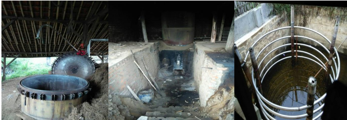
Figure 6. Process equipment of steam distillation used in H. Ede refinery
