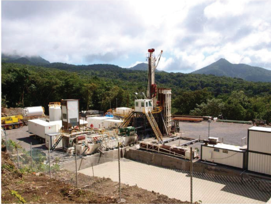
Figure 46 Rotary rig drilling slim holes up to 1500m (Source: ISOR)
