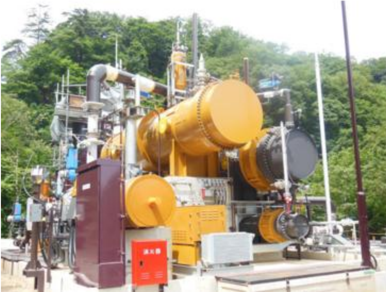
400-KW Onsen Binary Geothermal Power Plant at Tsuchiyu, Fukushima Prefecture, Credit: Genki Up Tsuchiyu Company
