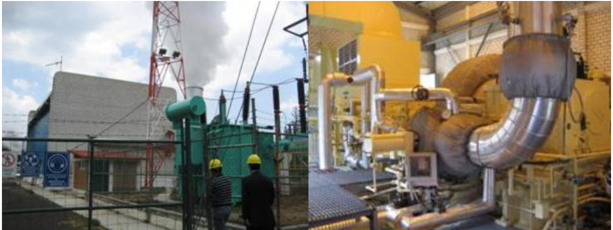
Figure 7: Well head generating unit small scale application in Los Azufres Unit 6 Mexico
