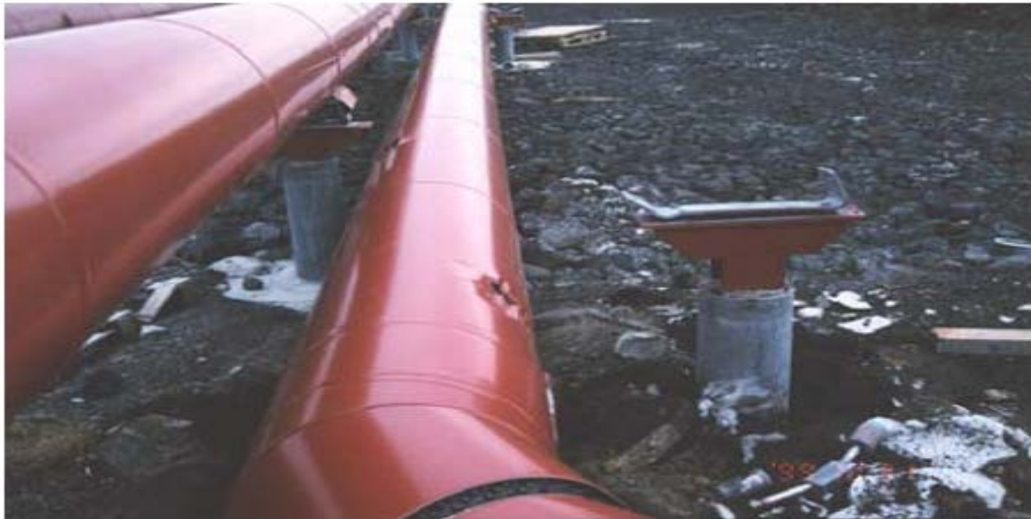
Figure 7: Slug flow knocked the pipe off its supports.
