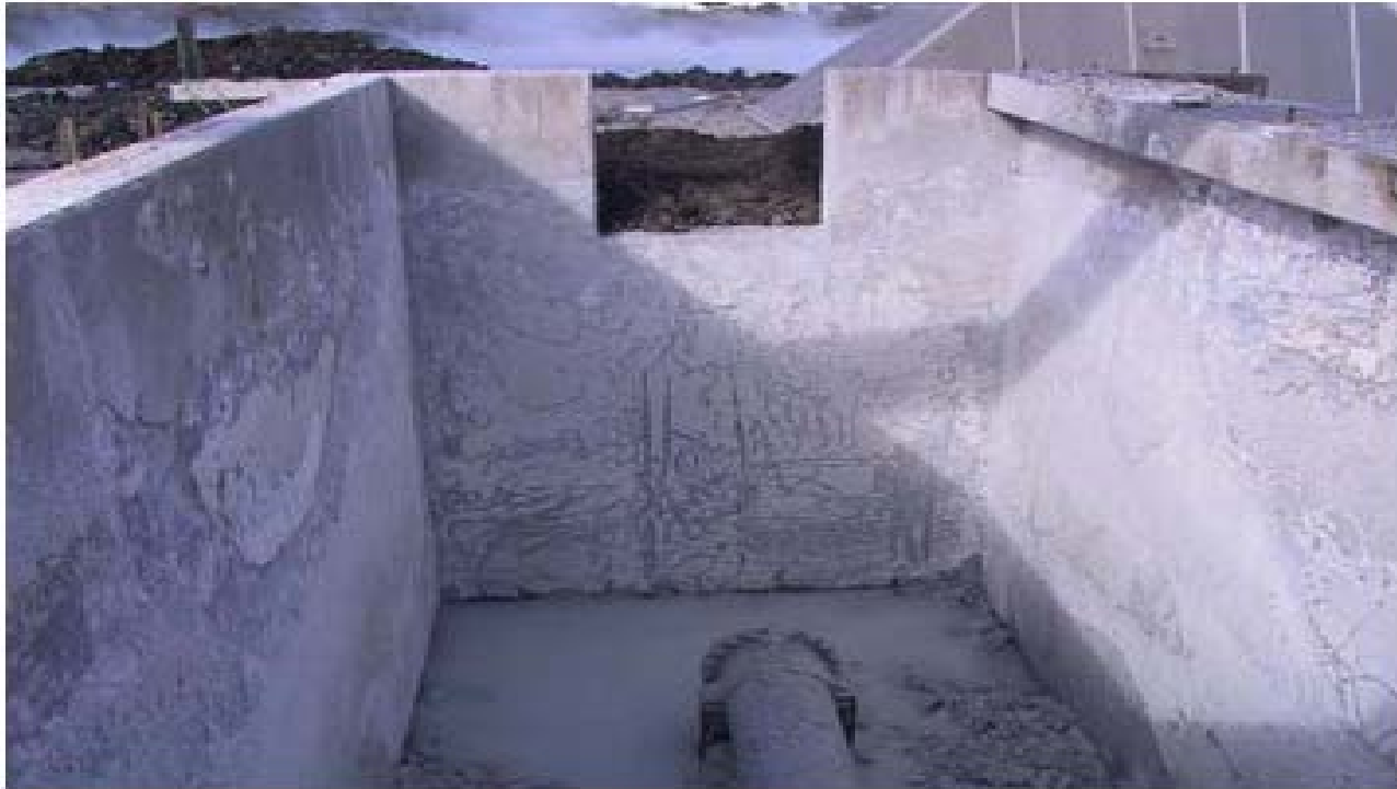
Figure 10: Silencer after cleaning. Inlet pipe can be seen on the bottom.
