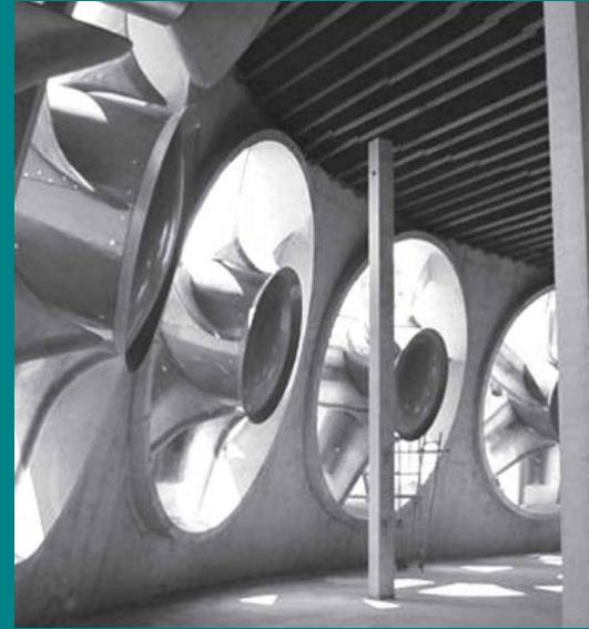
Inside of a Fan-assisted natural draft tower
