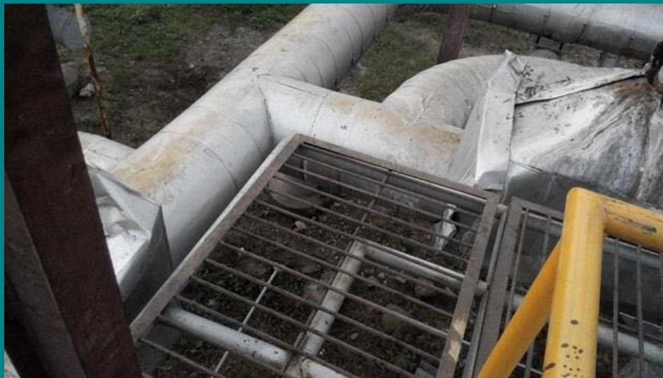
Substandard Platform & Grating
