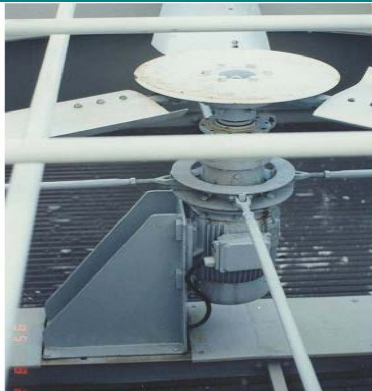
Figure 13: ORC cooling fan with gear motor.
