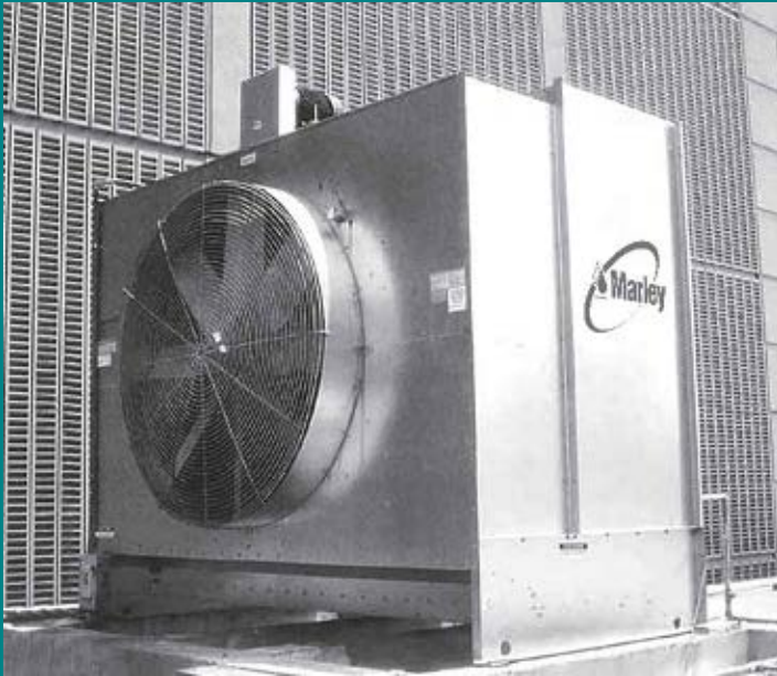
Small factory-assembled tower
