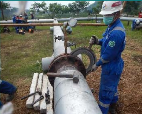
Orifice Inspection
